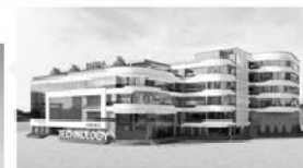
IDEA HI-TECH Saigon Hi-Tech Park, District 9, HCMC 14,500.25 m 2 | Block A - 3 Floors, Block B - 4 Floors, Block C - 5 Floors Project management | Supervision Consultants
