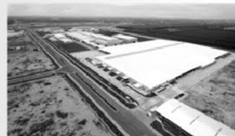
LIXIL GLOBAL VIETNAM FACTORY 01 Road, Long Duc Industrial Park, Long Thinh District, Dong Nai 58,100 m 2 | 6 Factories & Building 1 | Budget: 65 mil USD Project manager | Kajima Viet Nam
