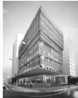
M BUILDING Phu My Hung, Tân Phú Ward, District 7, HCMC 9,218 m 2 | 19 Floors & Basement Project management | Supervision Consultants
