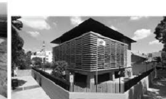
CONSULATE GENERAL OF JAPAN IN HCM CITY 281 Dien Bien Phu Street, District 3, HCMC City Construction manager | Kajima Viet Nam
