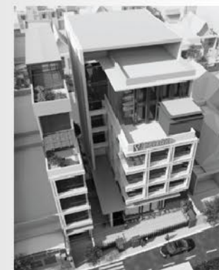
AB TOWER Esuhai School Aop Bac, Tân Bình District HCMC Supervision Consultants
